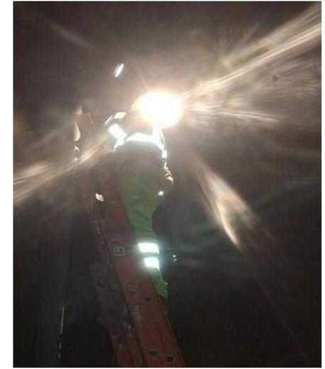
REEMPLAZO DE FOCO Y BALASTRO, SE RECONECTA LÁMPARA
